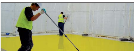
Blue Applying a floor coating system
